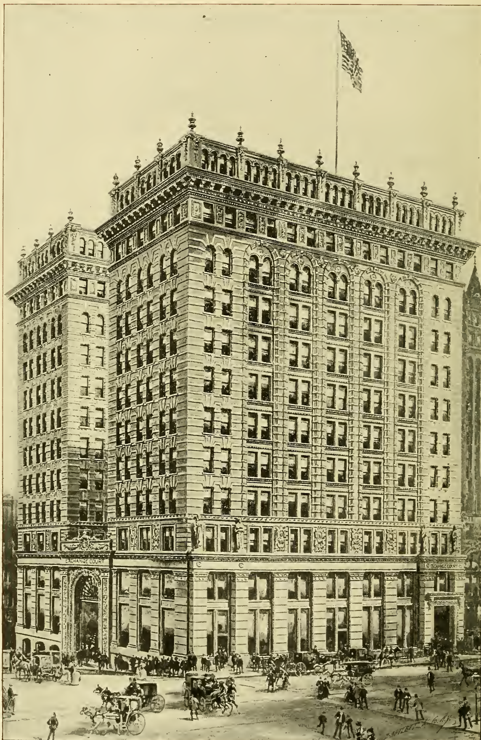
Exchange Court Building, New York. 632 H.P. Babcock & Wilcox Boilers.
